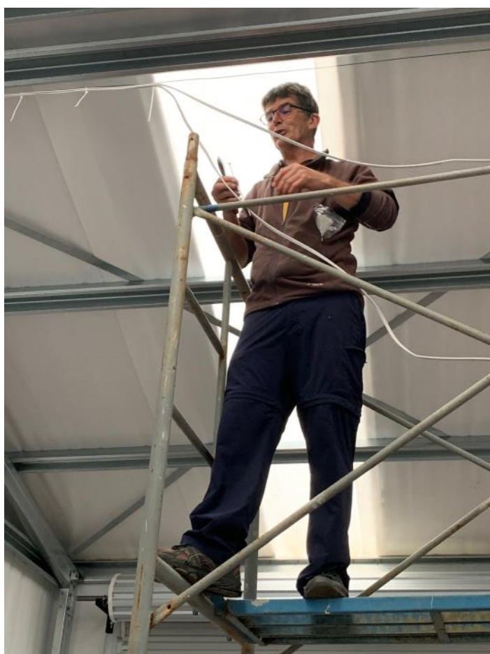
Gary Learmonth installs lighting cables in the new shed
