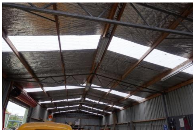
New skylights in the restoration shed
