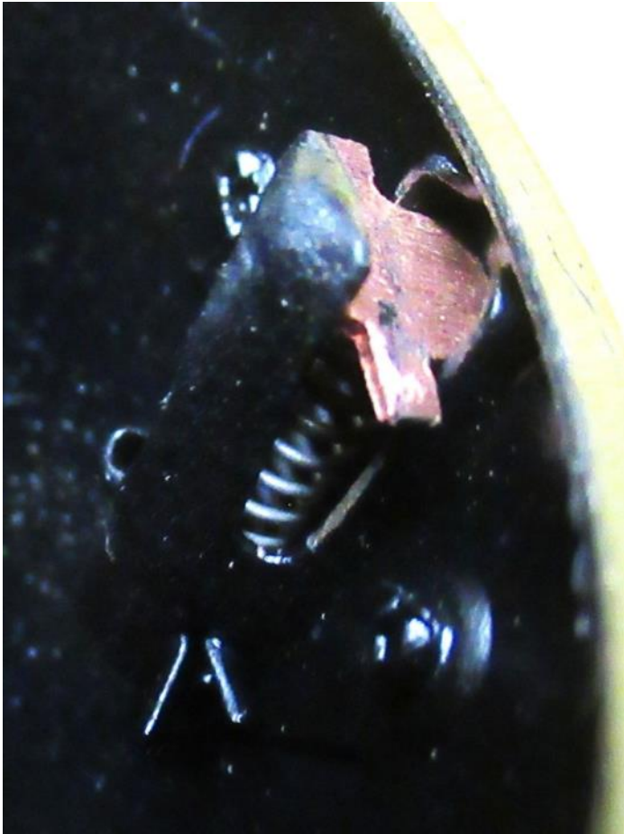
Copper washer and spring to hold reflector and glass in position.
