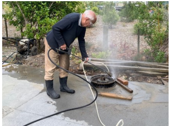
Water Blasting the BSA wheels.
