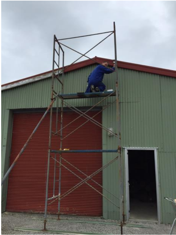
Coxy up the scaffold.
