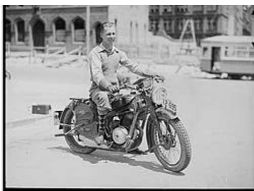
Rider on a Coventry-Eagle in, Australia, circa 1935. The machine has a pressed steel frame; Villiers two-stroke engine; and twin exhausts.
