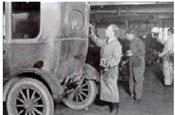
This 1923 photo shows Charles Jeffery, an instructor at Master Motors Coach Refinishing of Detroit, using the latest technology in auto refinishing: paint brushes. Back then, cars were sanded with gasoline between brush-painted coats and polished with emery cloth. (Photo courtesy of PPG.)
