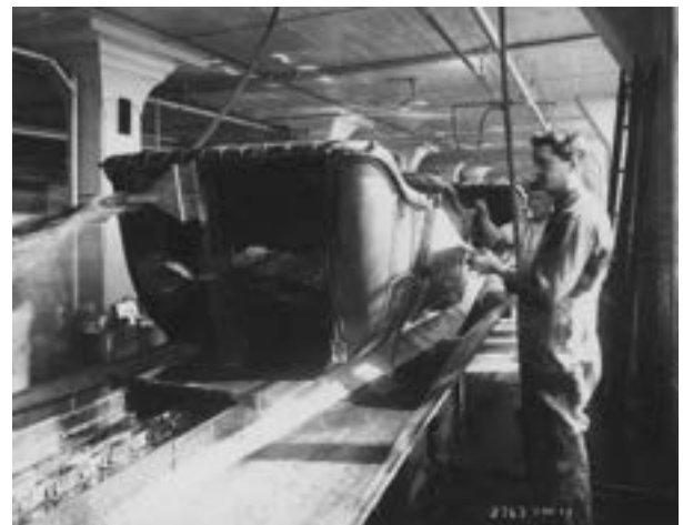
This 1923 photo shows Charles Jeffery, an instructor at Master Motors Coach Refinishing of Detroit, using the latest technology in auto refinishing: paint brushes. Back then, cars were sanded with gasoline between brush-painted coats and polished with emery cloth. (Photo courtesy of PPG.)
